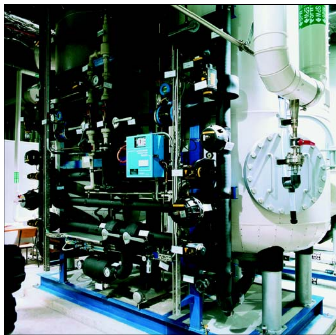
Figure 3. Softeners in series.
