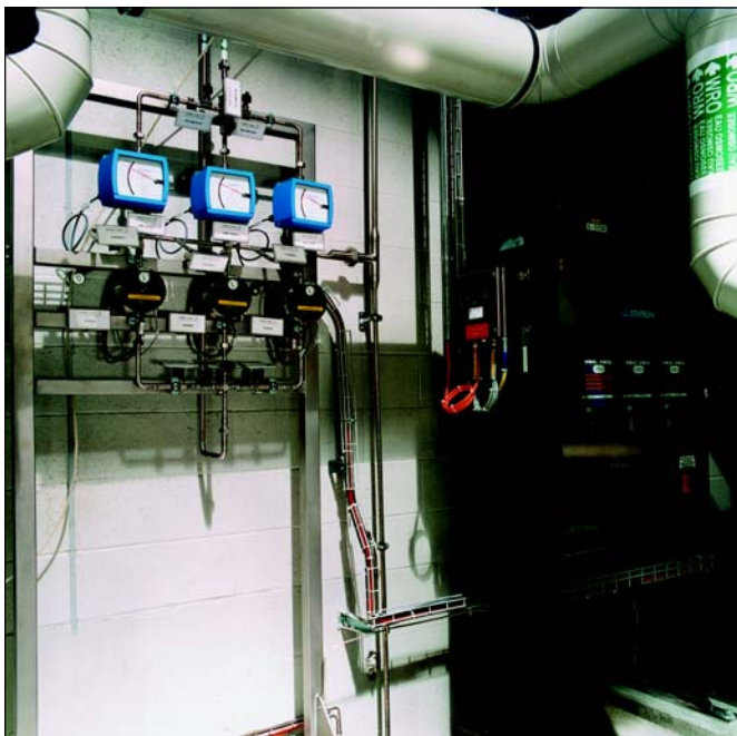
Figure 5. Ozonization plant (3 x 4 gO 3 /h).
