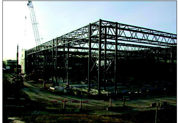
At this stage in construction, piping in the basement was already completed.
