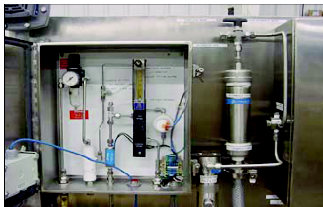
Figure 3. O 2 sampling panel.
